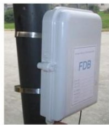
FTTH-005 fiber termination box on the pole
