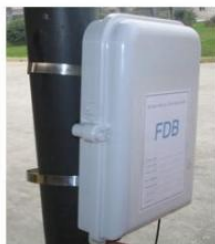
FTTH-005 fiber termination box on the pole
