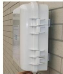
FTTH-005 fiber termination box on the wall
