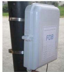
FTTH-005 fiber termination box on the pole
